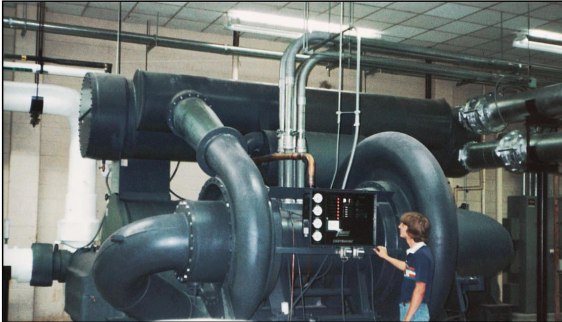
Reducing CHS temperature penalizes chiller efficiency but can save pumping power.
